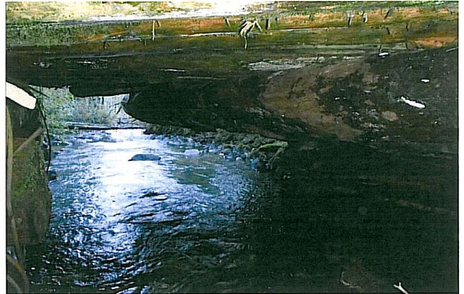
CK-2346 Stringers and left abutment
